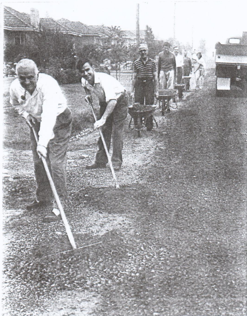
Settling In Spreading Road Metal
